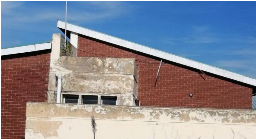
DAMAGES CEILINGS AND SHOWER WALLS AT COUSIN SENATLE
