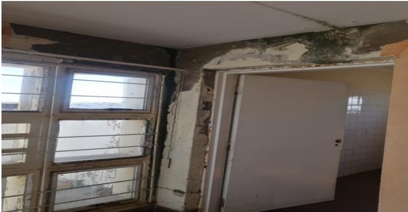
LEAKING ROOF AT RESIDENCE
