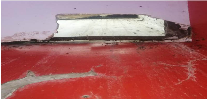
LEAKING ROOF MAIN HALL AFFECTING BRICKS
