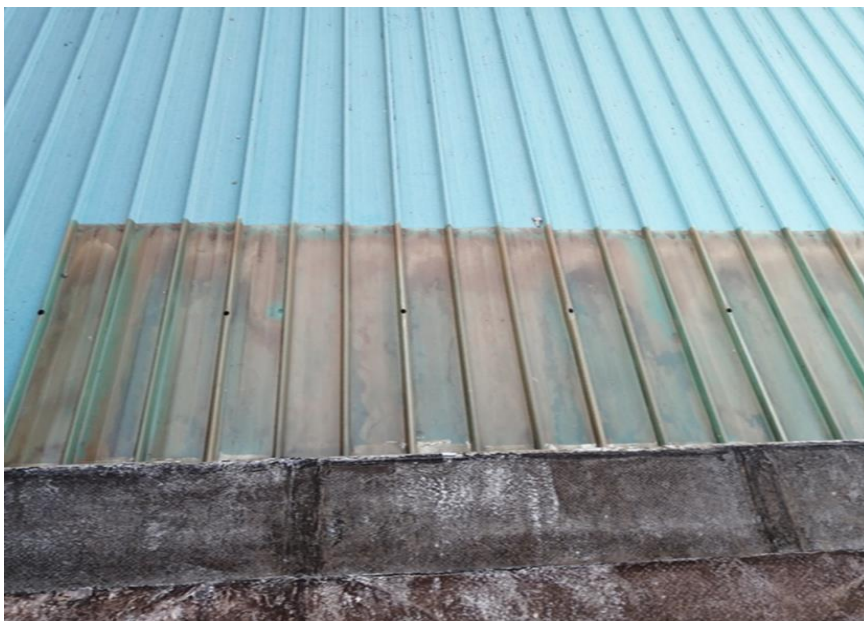
LEAKING ROOF MAIN HALL
